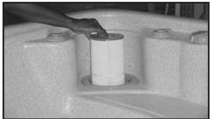
4. Remove filter cartridge and wash it with a garden hose inside and out until the cartridge is clean. Reinsert the filter and follow the steps in the reverse sequence.
